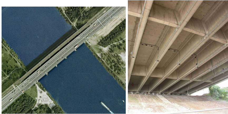
Fig. 1. (left) Aerial picture of the situation of the Hollandse Brug, which connects the ‘island’ Flevoland to the province Noord-Holland, and the adjacent railway bridge (top). (right) Some of the sensors attached to the underside of the bridge.
